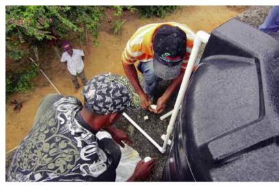
**Photo:** Last August, we installed a water filter on the roof of the elementary school in the village of Los Cerezos, in the heart of the Tree Bank project area. The filter provides students and staff with a source of parasite-free drinking water. The water itself comes from our new park, which protects the origins of the streams that flow into the village. The park helps guarantee the village water supply.
