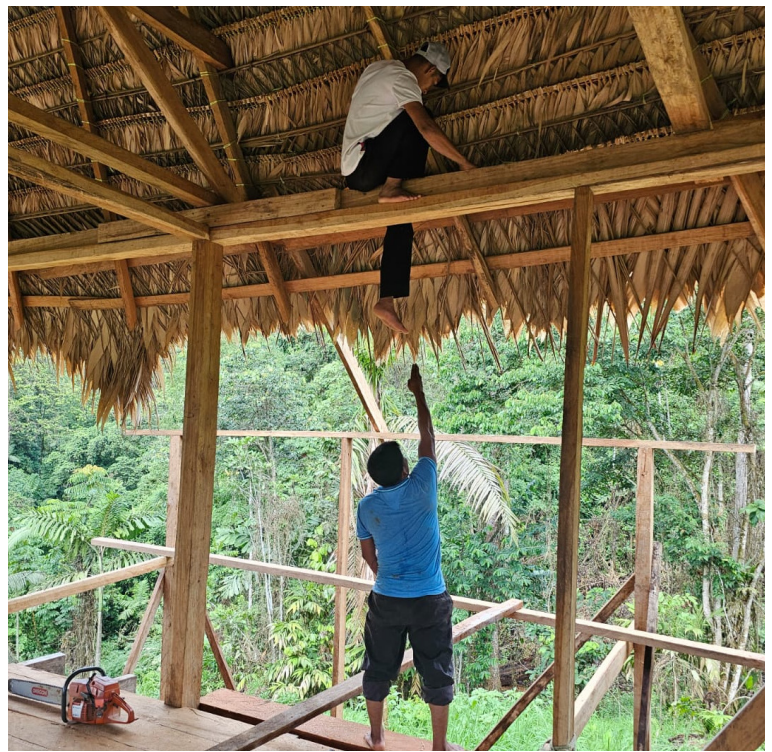
Above right: In our Panamanian rainforest site in September, our crew installed a traditional Naso roof on our casa de vigilancia . The activity has already spooked the local poachers, and some wildlife is returning.
